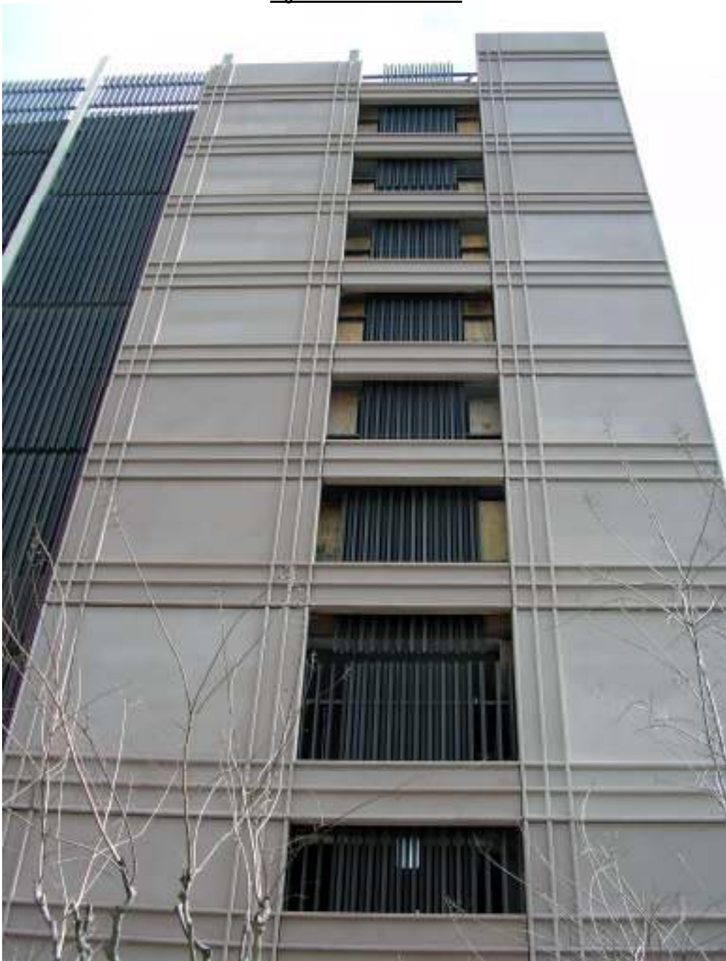
Fig. 4: New GFRC Facade
