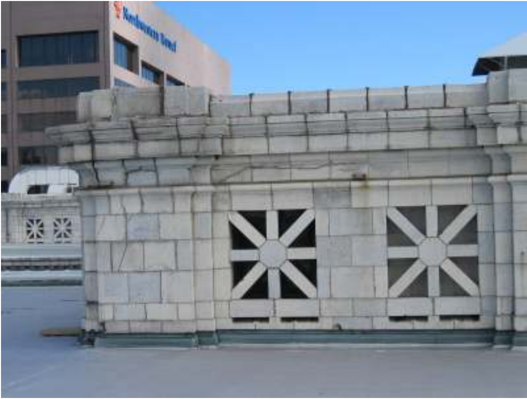
Fig. 1a: Terra cotta Penthouse (Before demolition)
