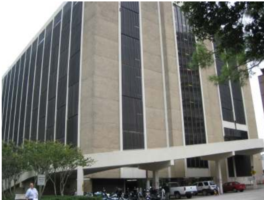
Fig. 3: Marblecrete facade before demolition
