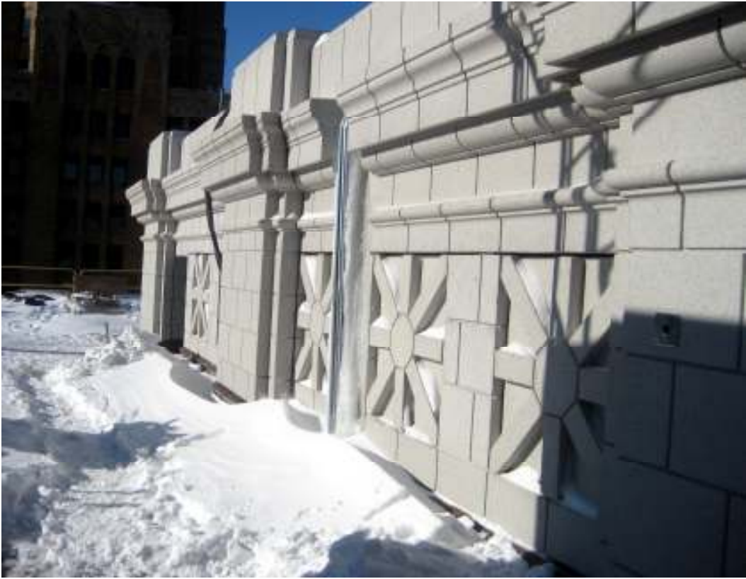
Fig. 1b: GFRC Penthouse (After recladding)
